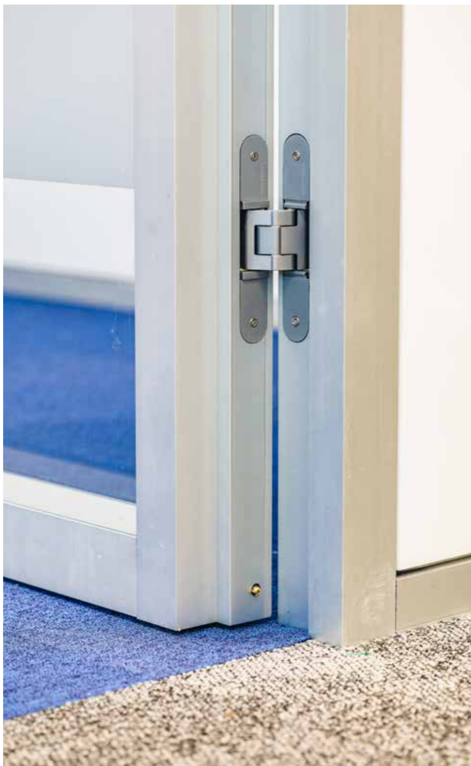
cerniera a scomparsa concealed hinge
